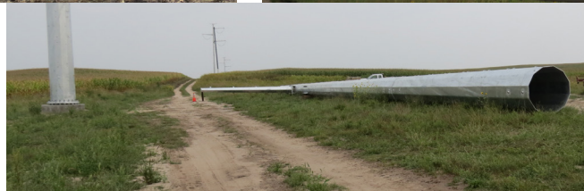
Clockwise from upper left - board members from left to right, Rod Zohner, Joe Thiele, Greg Weidner, Dennis Kuchar and Mark Miller attended the tour; setting a structure on a base; structure staged on ground for setting; foundation being jacked and framed ready for concrete.
