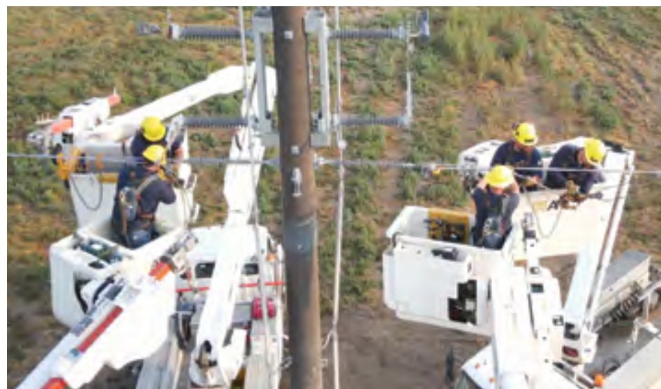
Pictured above: Crews work on a line build project.
