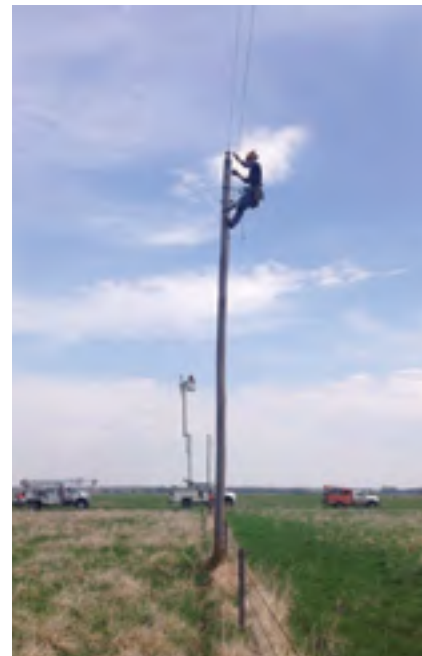
Crews working to repair damage to the lines after a storm.
