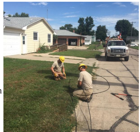
Crew working in Elgin stringing new wire.
