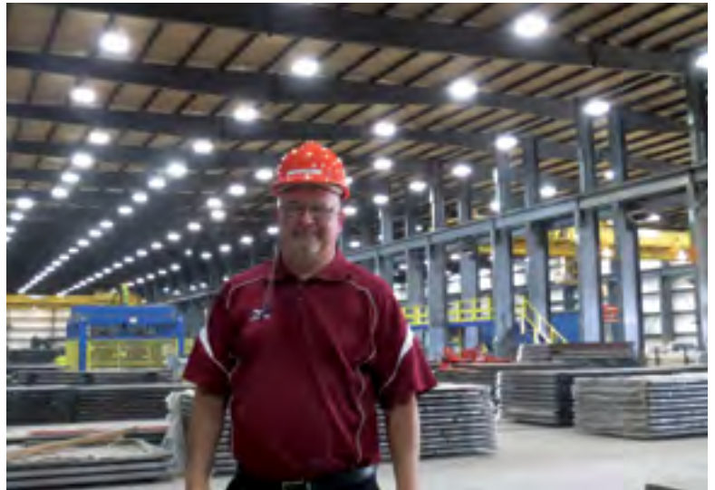
Scott Orwig, Corporate Facilities Manager for Norfolk Iron and Metal, shows off some of the 866 light fixtures that were upgraded to LEDs. This will save NIM 1,532,404 kWh and $70,050 per year on their electric bill. This is a Public Power Advantage.
