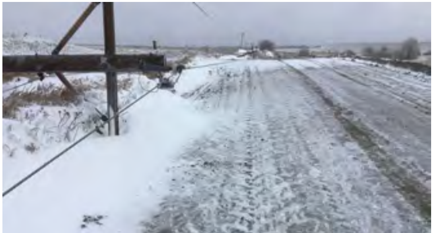
Pictured above are poles down in Madison County north of Newman Grove during the ice storm at the end of March.
