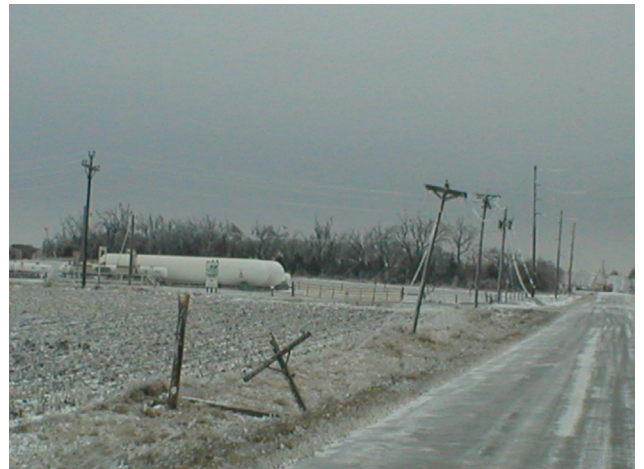
Ice Storm Damage 2006
