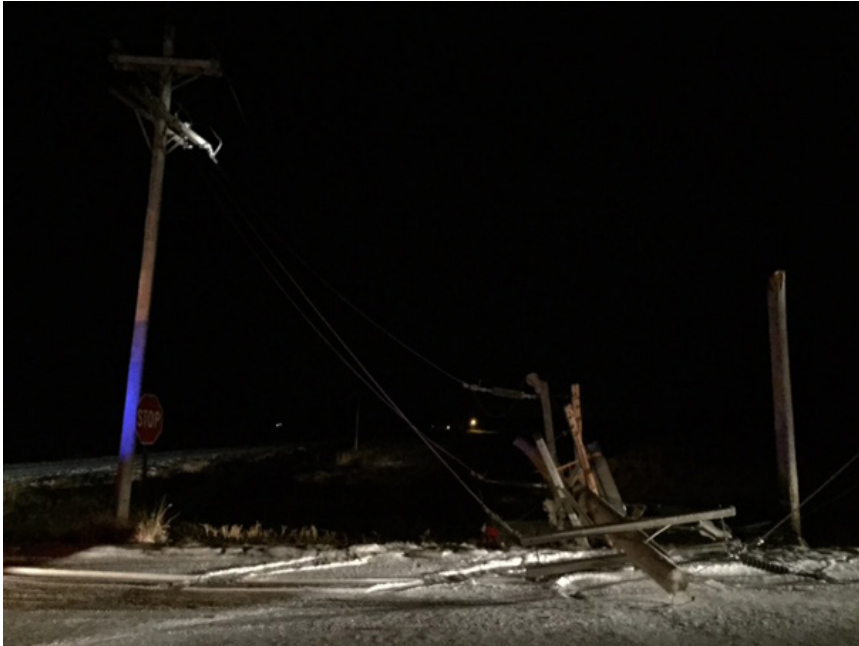
November accident scene at the intersection of South First Street and Sherwood Road.
