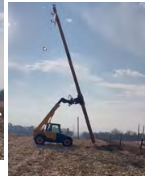
Utilizing smaller equipment, like a telehandler, saves crews time and wear and tear on larger more expensive equipment like a digger derrick. While not for every situation, having this equipment gives crews a lot of flexibility in how to do the work, like setting poles - pictured here.
