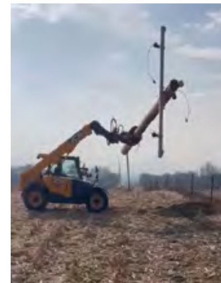
Utilizing smaller equipment, like a telehandler, saves crews time and wear and tear on larger more expensive equipment like a digger derrick. While not for every situation, having this equipment gives crews a lot of flexibility in how to do the work, like setting poles - pictured here.
