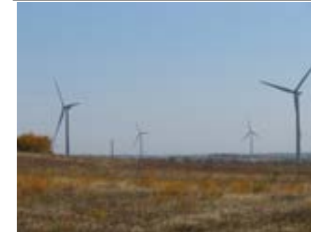
Above: Some of the first wind generators erected for the Prairie Breeze projects.
