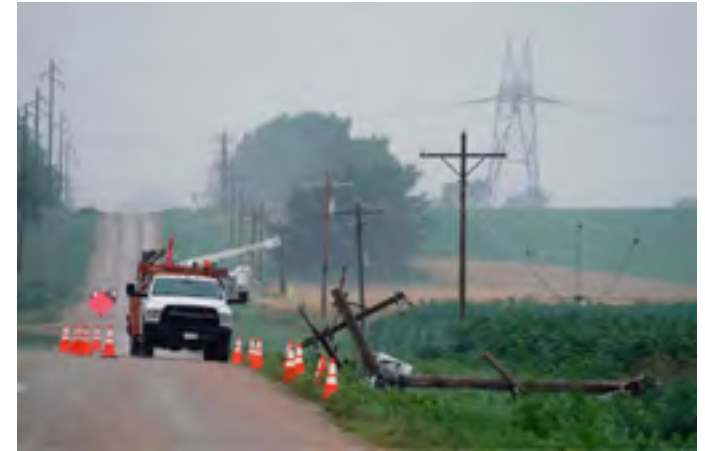
Neligh crews are fixing a pole and line that was damaged during a storm in the Summerland area on July 16, 2022. The use of signs and cones warn drivers to slow down and proceed with caution through the work zone. (Photo courtesy of the Antelope County News Facebook page.)
