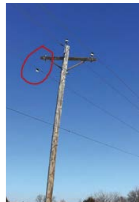
Pictured above – transformer bracket broken and transformer hanging by the jumper. Pictured below left to right - 69 kV switch opened and arcing due to the destructive galloping of the line (picture from video taken by Keith Heitoff ); broken cross arm and insulator has been shaken off the pole.
