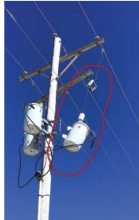
Pictured above – transformer bracket broken and transformer hanging by the jumper. Pictured below left to right - 69 kV switch opened and arcing due to the destructive galloping of the line (picture from video taken by Keith Heitoff ); broken cross arm and insulator has been shaken off the pole.
